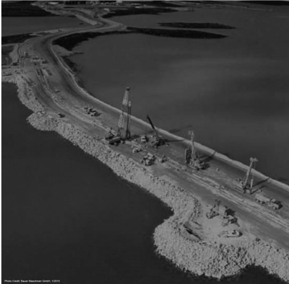
Figure 7-4 – Example of Slurry Wall Construction-Diavik Diamond Mine
